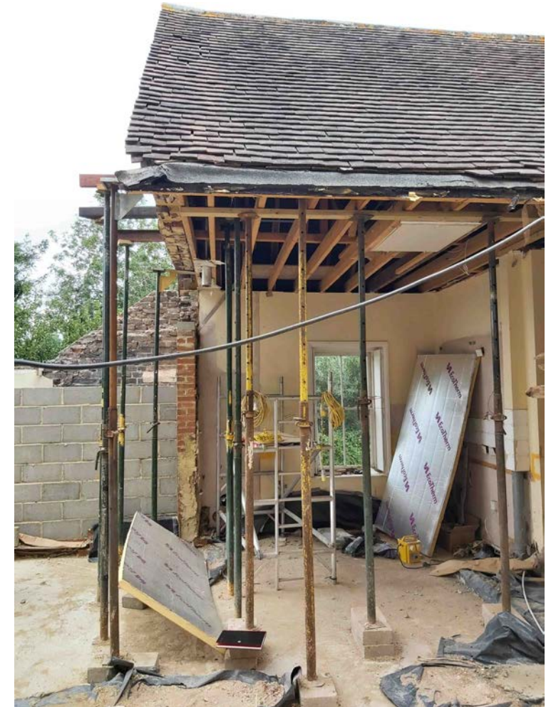
A concealed steel beam enables the space under the stable roof to become part of the continuous open plan kitchen area
