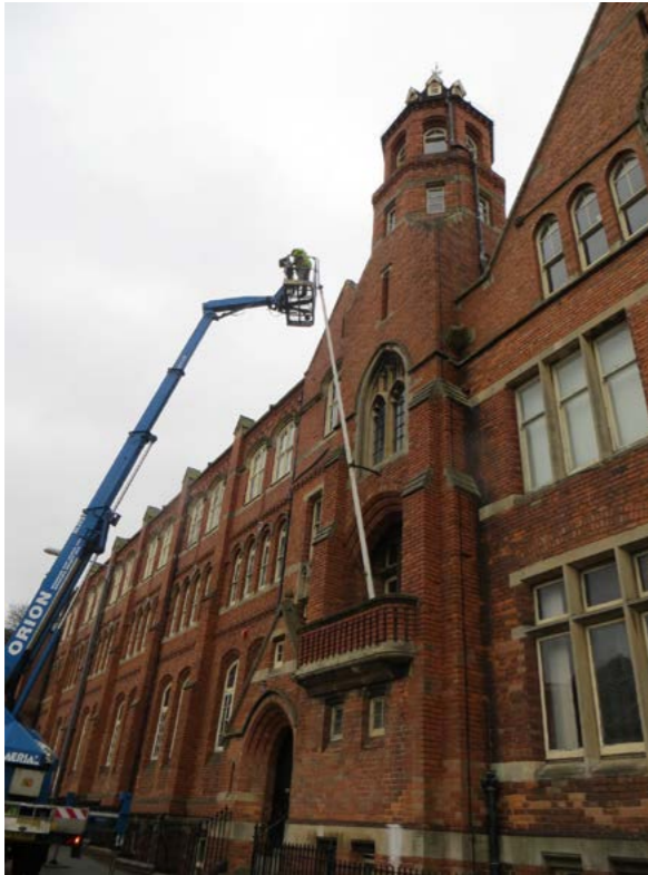
Roof survey and inspection
