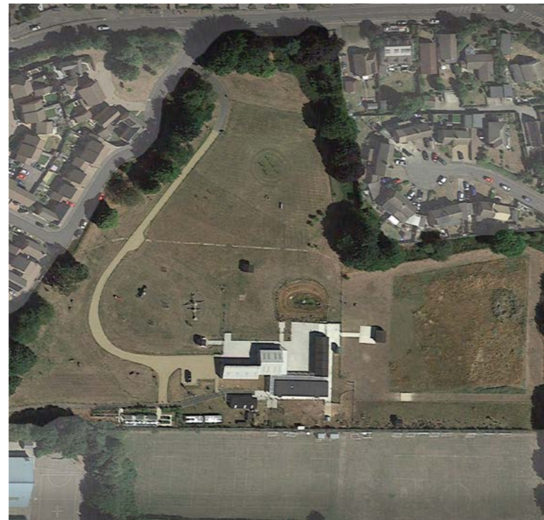
Aerial view of the completed Rural Activities Centre
