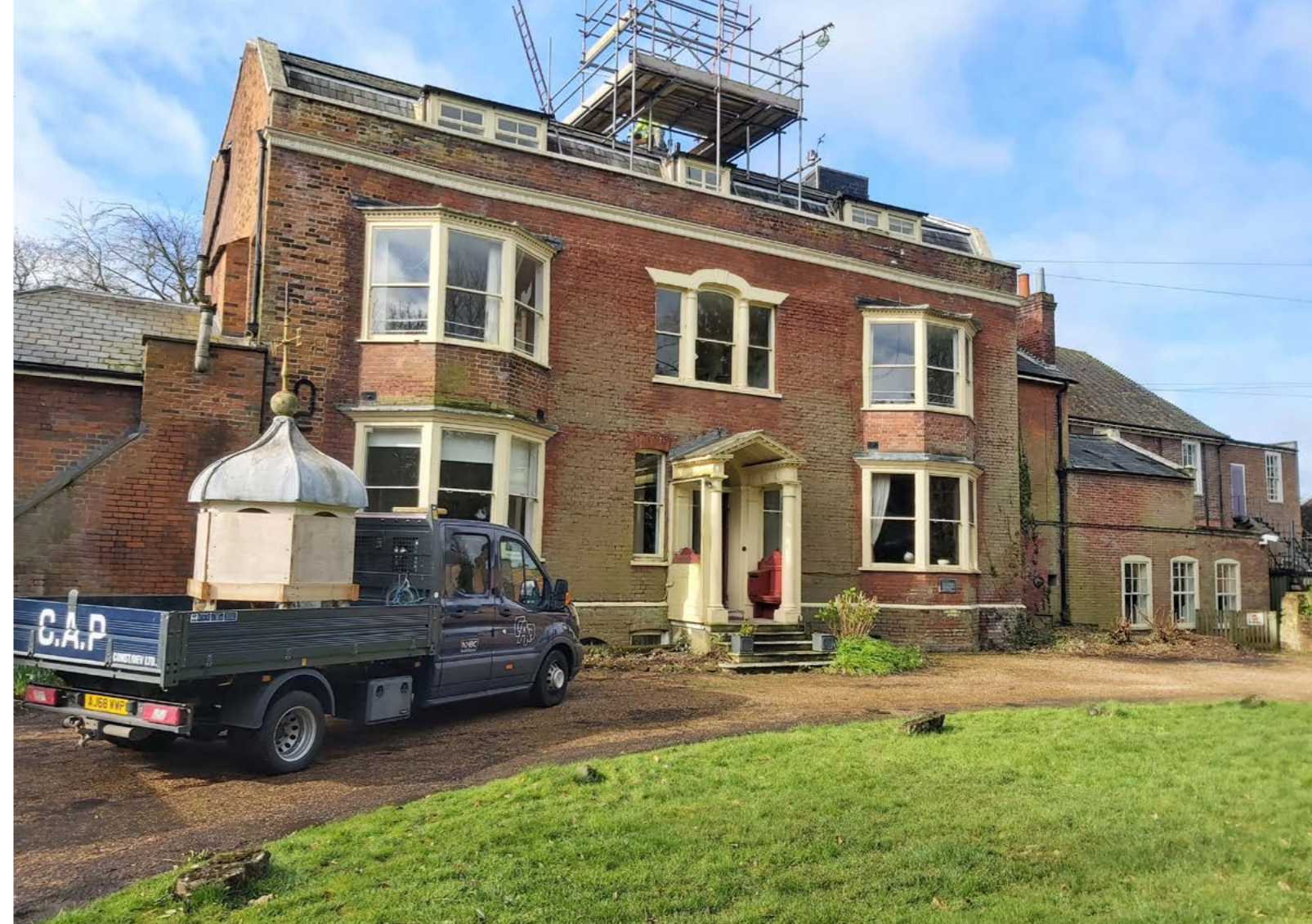
Removal of cupola at Gad's Hill Place for refurbishment
